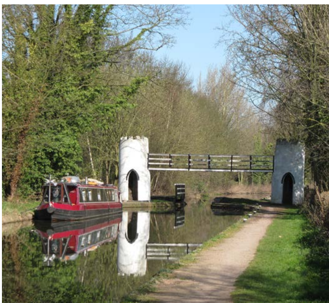
Drayton Turret Bridge on the Birmingham & Fazeley Canal. © Kate Sugden (WWT) 2015.
